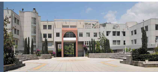
HYATT PLACE HOTEL Hotel Uyo - Nigeria
